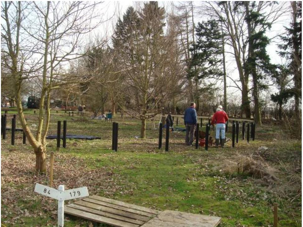
Work is now underway again on the new "G1" track. In the foreground Matt Stallard, David Wesy & Norman Back are busy filling the pipe with concrete and setting the top studding. Geoff Mogg is at the back checking laser levels are correct.
