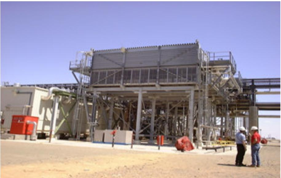
*A high pressure gas cooler installed at site*
