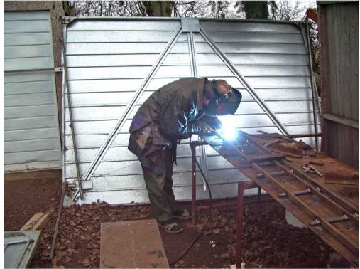
*Mike Hodgson MIG-welding fishplates on to the ends of a panel. According to Mike, doing all the welds on a 20ft panel consumes 10 feet of the filler rod.*
