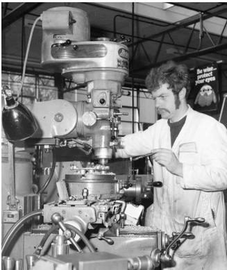
*Any general consideration of the varieties of milling machines had to include reference to the Bridgeport Series 1 milling machine. Mike included this picture of one such machine once housed in the main workshop at St. Albans College and seen here being used by Ray Baskerville.*
