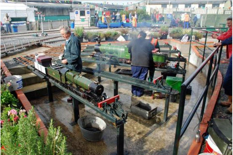
East Somerset SMEE members built this radial style sunken steaming bay facility in just one winter. Three steps lead down from ground level, a fine turntable links the bays to the main line and a sturdy barrier provides comfort for onlookers.
